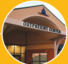
The Christ Hospital Outpatient Center - Anderson 7545 Beechmont Ave. Cincinnati, OH
